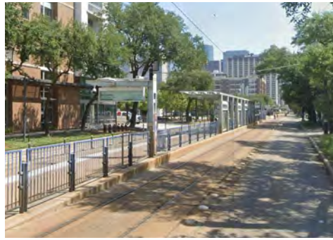
METRO RAIL STOP | MCGOWEN
