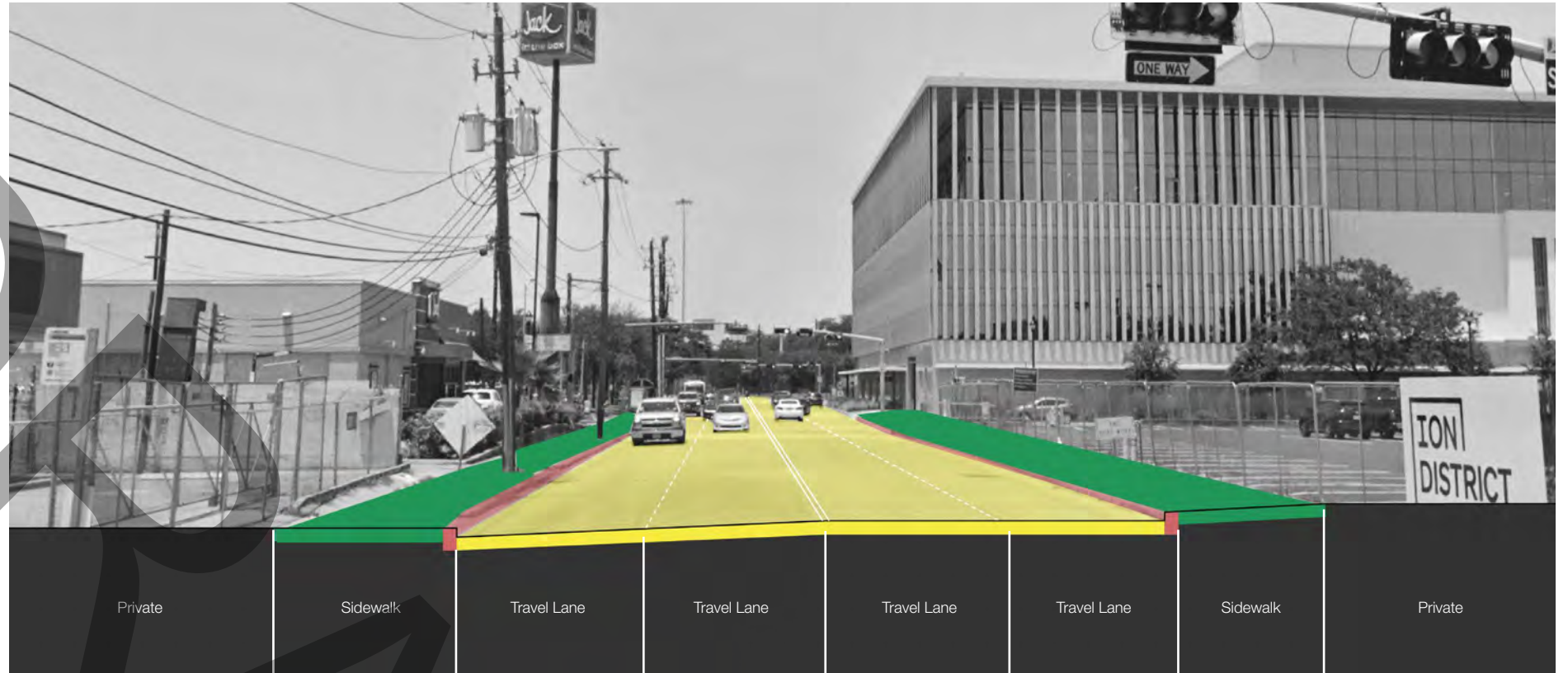
Figure 47 Existing Street Conditions
